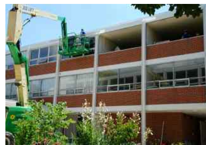
New windows were installed in Deming Hall and Lovett Hall, among many other renovations completed across campus this summer.
